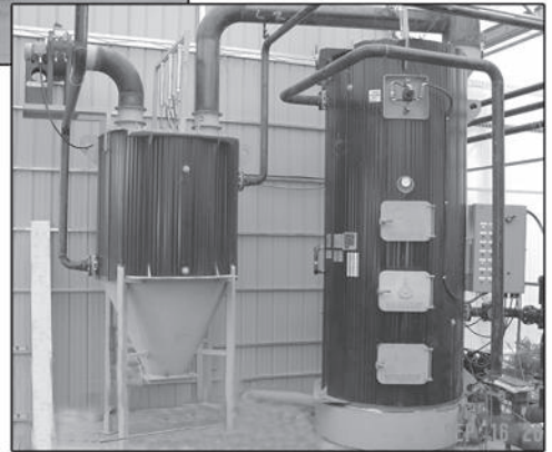
Eliminate fly ash and improve efficiency with a waste heat exchanger (left). Use with any new or existing Decker boiler.
